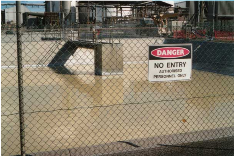
Storm water pond containing 10% acid and a high dissolved metal content.
